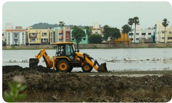
Photo showing dredging operations at Sembakkam Lake
