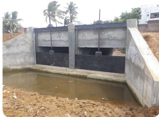
After construction of flood regulator gates in May 2019
