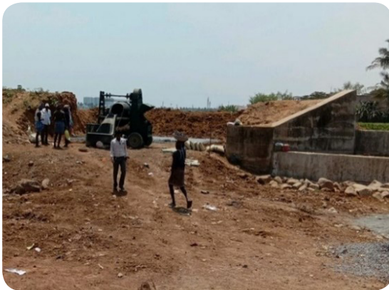
Before construction of flood regulator gates
