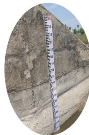
Staff gauge installed at the surplus weir of the Sembakkam Lake for measuring water levels
